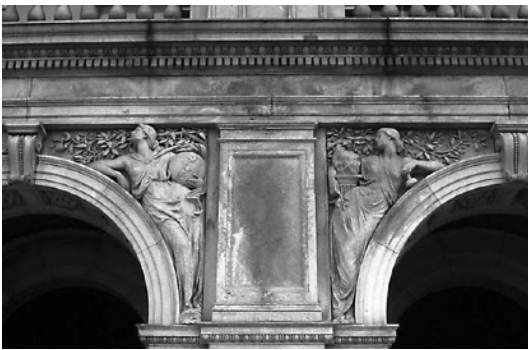
Figure 2. Two spandrels, decorated with allegorical figures. The spandrel space is a consequence of the firmitas of the arch, as the chosen means of supporting the horizontal architrave between columns to make the utilitas of the functional opening.
